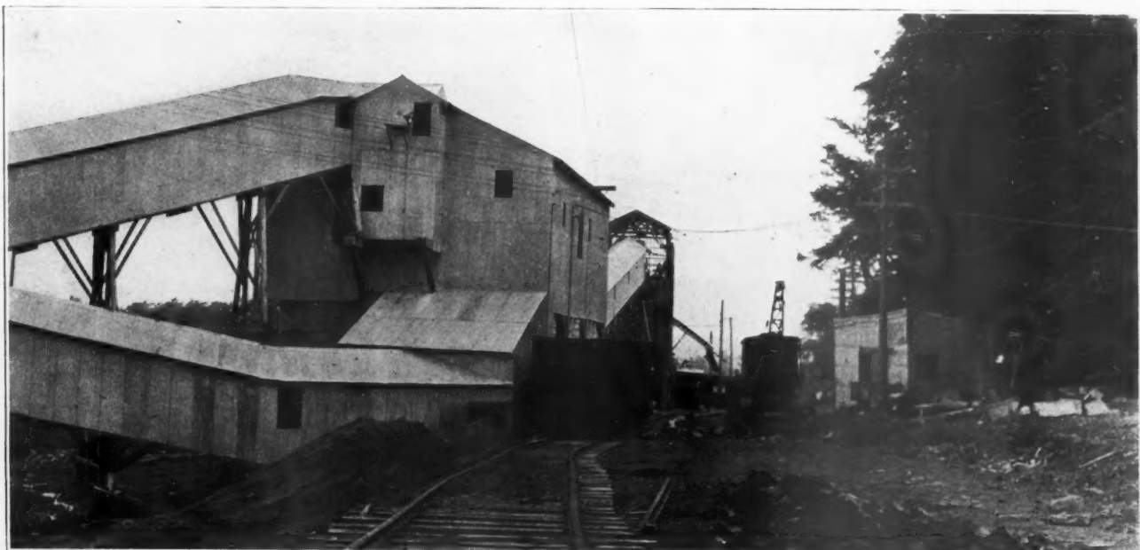
View of Screening Plant Showing Conveyor from the Crushers, Return Conveyor and the Conveyor to the Lime Plant in the Background. Also Freight Car Dumping Load Into Hopper Under Tracks.
